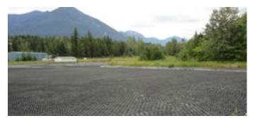
"Familiar with the Hexa-Cover<sup>®</sup> Floating Cover, I felt the product could nicely cover the lagoon, controlling the algae growth as the sunlight would not be able to penetrate into the water. Additionally, the Hexa-Cover<sup>®</sup> Floating Cover would enable the aeration process and fluctuating water levels to continue"
