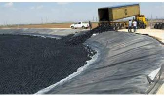
Hexa-Cover<sup>®</sup> Also installation in empty tank (max 5m drop)
