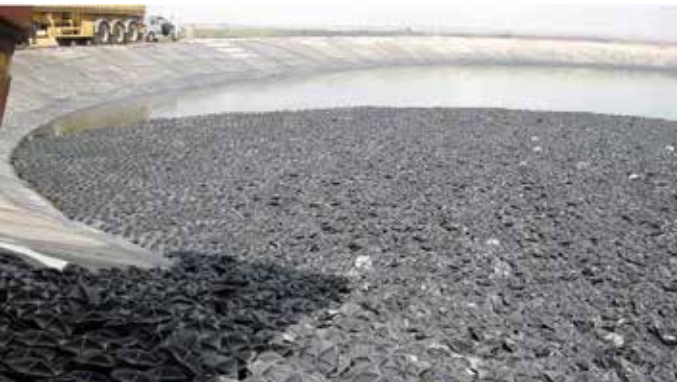
Hexa-Cover® Floating Cover BULK delivery and installation:
